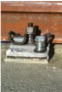
Support after concrete pouring
