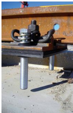
Clipped components before concrete pouring
