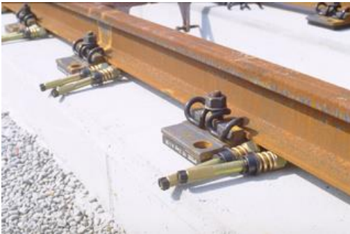
Bottom-up construction method
