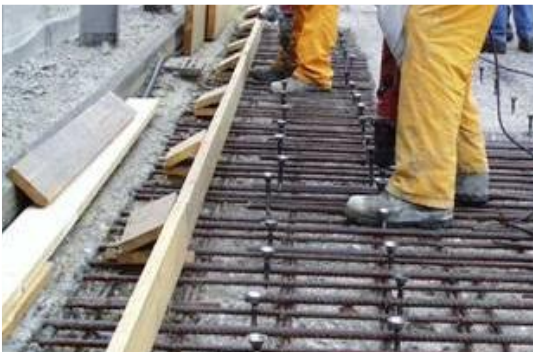
Slab strengthening
