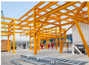
a) Primary steel column
