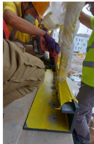
c) Placement of steel profile
