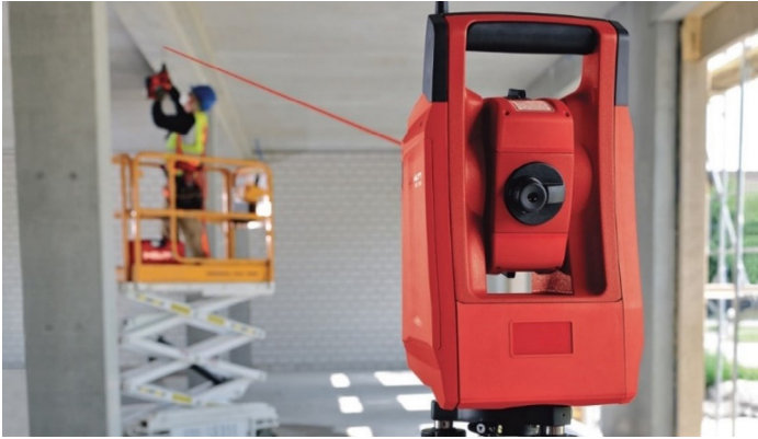
Fig. 8.4: Use of laser at a jobsite while positioning bore holes
