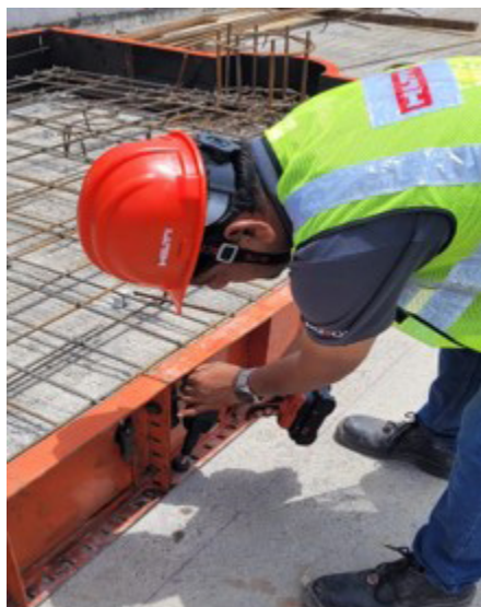
a) Baseplate / Shutter frame fixing application during construction
