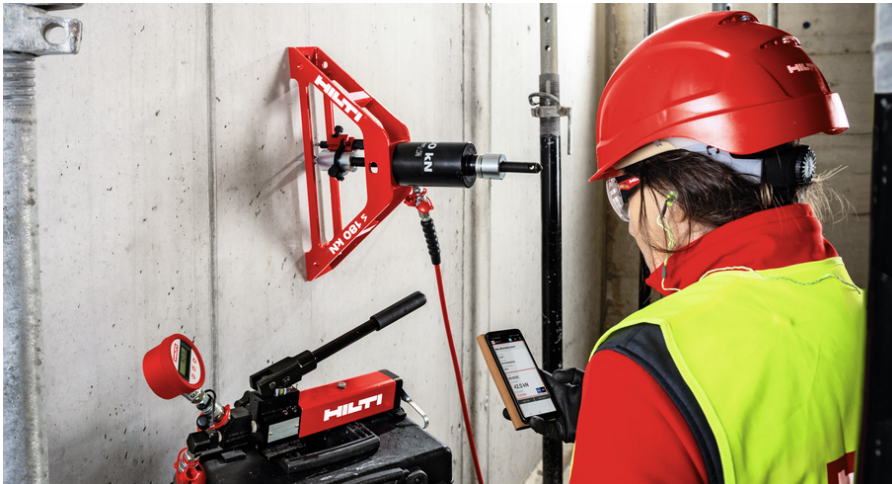
Fig. 8.19: Onsite testing by Hilti (unconfined tension setup)
