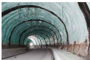
a) Road tunnels are highly corrosive environments
