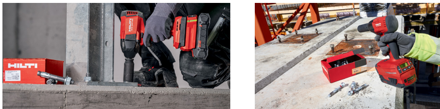
Fig. 8.16: SIW system torque wrench and AT module
