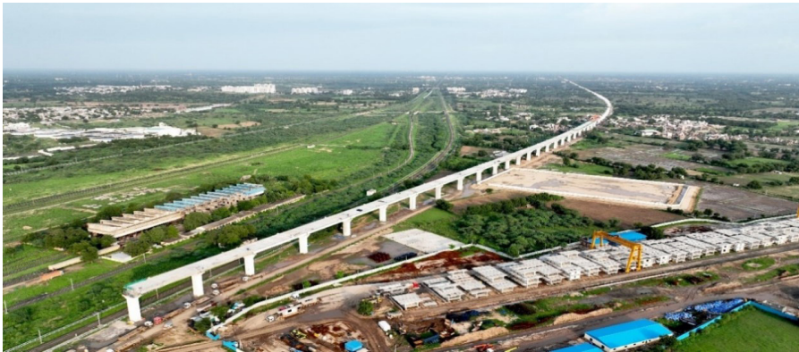
a) MAHSR viaduct portion
