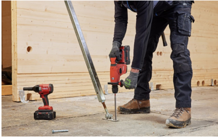
a) Drilling holes with a Rotary hammer
