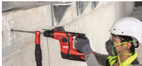
b) Drilling being done for horizontal application
