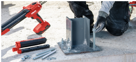
a) Anchors installed in vertically downward direction
