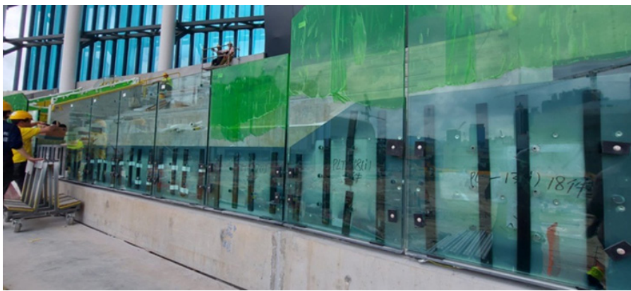
a) The structure at job site
